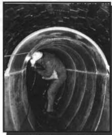
Sewer rehabilitation can include lining aging sewers (photo: NJ Department of Environmental Protection).
