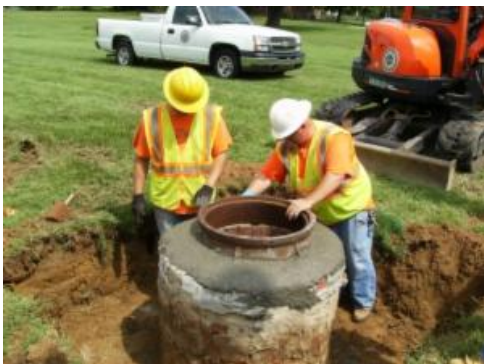
Manhole Repair
